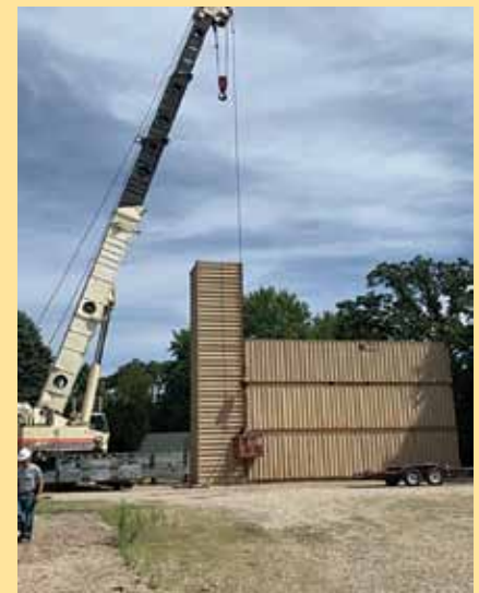
Construction underway on education and training building
