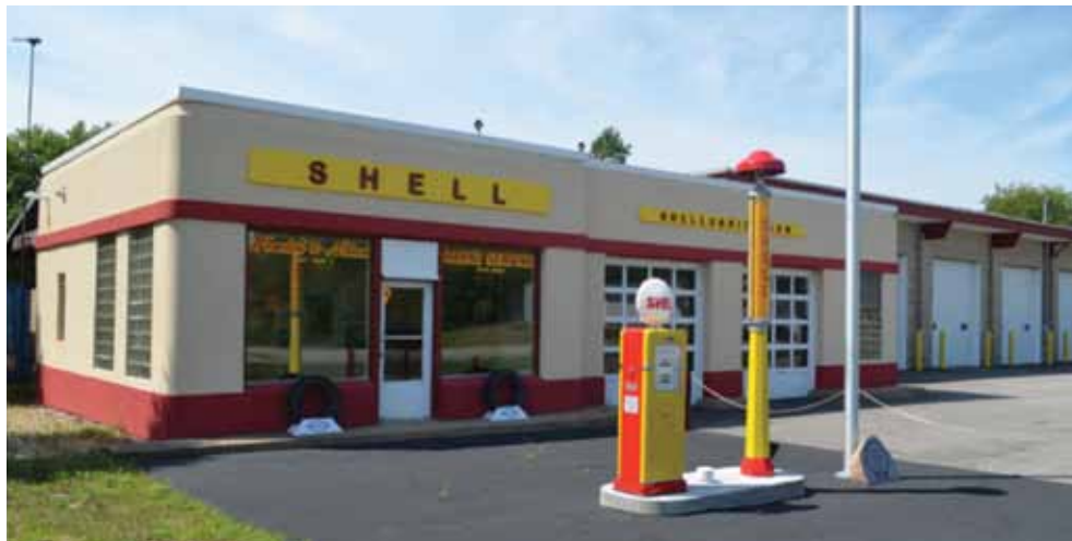
Left: History on display outside and inside our new Maintenance Building.
