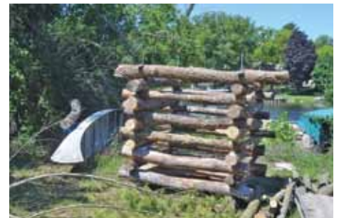
Larger "log cabin" cribs LLIA has been building and placing for years
