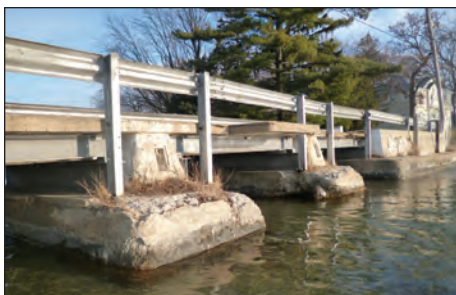
The Deakin Isle bridge that will be replaced this fall.
