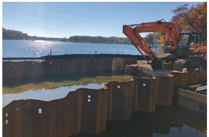
Construction of the new bridge structure underway. All photos this page by Patty Hargrave
