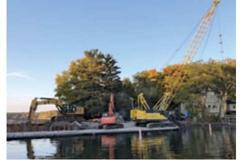
A view of the construction site from Middle Lake.
