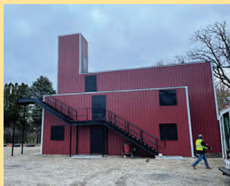
New training center as it looks now painted, completely enclosed, and nearly ready for lots of training.
